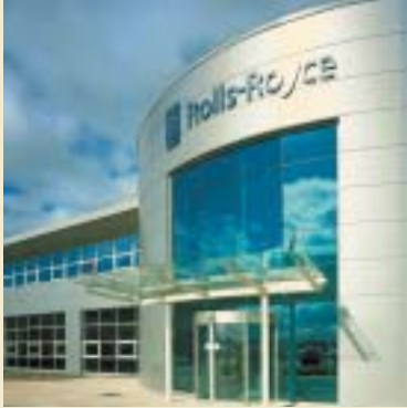
Project: Rolls-Royce Aerospace Location: Glasgow, United Kingdom Architect: Bradford Robertson Architects
